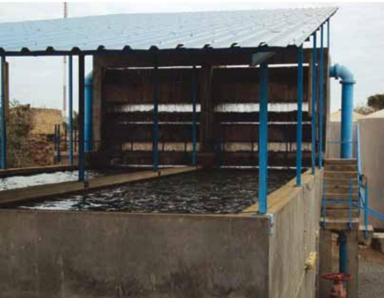
Water treatment by aeration process for iron removal - Tete.
