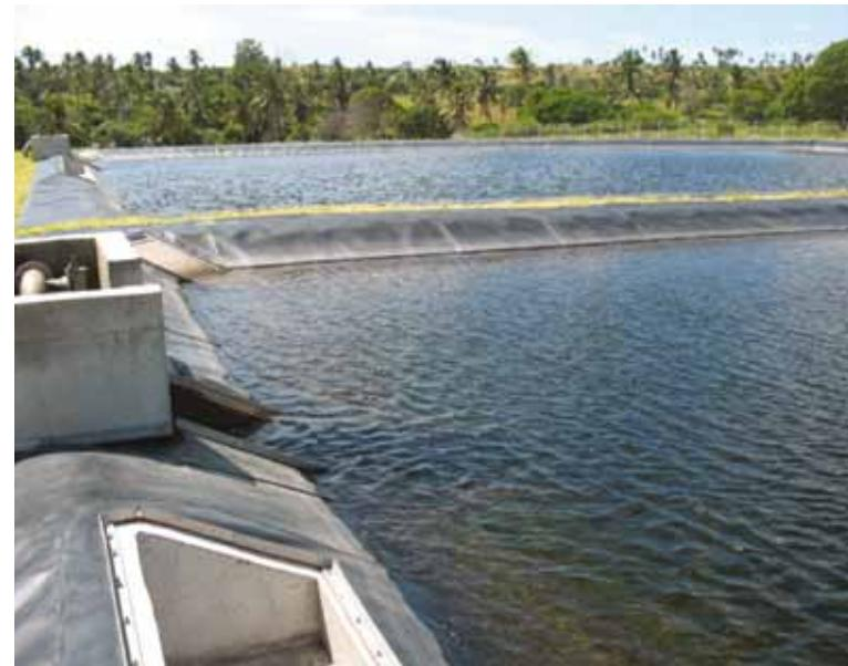
Water treatment process through slow sand filtration in Inhambane.
